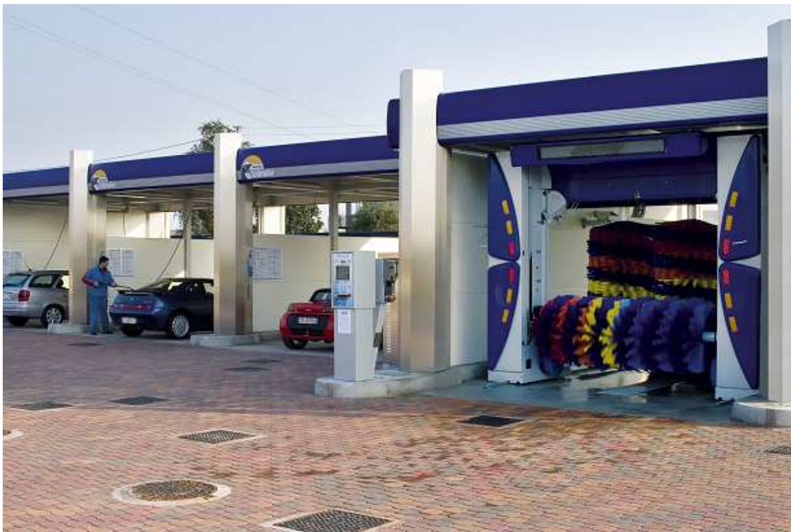
Many operators include an automated car wash to increase site capacity. The Ceccato Hydrus shown here washes up to 14 cars per hour.
